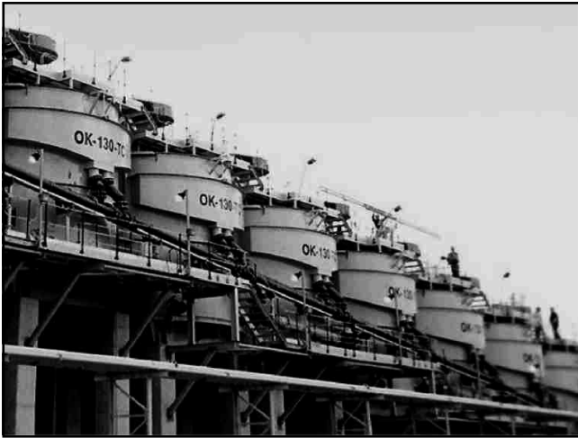
Figure 3. Tank cell installation.
