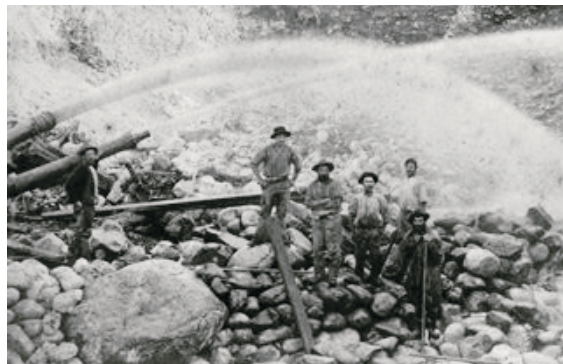
Gold sluicing at Kumara, West Coast, South Island in the 1880s/Alexander Turnbull Library
