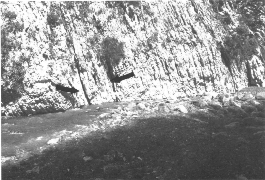
Plate 2: Haumurian Limestone and Teredo Limestone (Units A and F), Muzzle Stream. Teredo Limestone forms slight ridge, extreme right. Arrows indicate two clefts, formed by soft marl marker beds, just left of centre.
