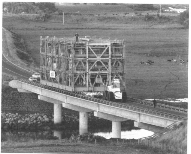
Plate 3. Plant relocated to the Motunui site.
