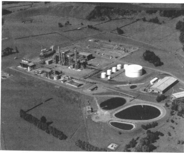
Plate 1. The 500 000 MT Waitara Valley methanol plant.
