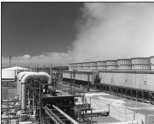
With 18 cells, the largest cooling tower in the southern hemisphere at Methanex's Motunui plant.
