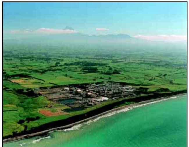
Methanol plant at Motunui.
