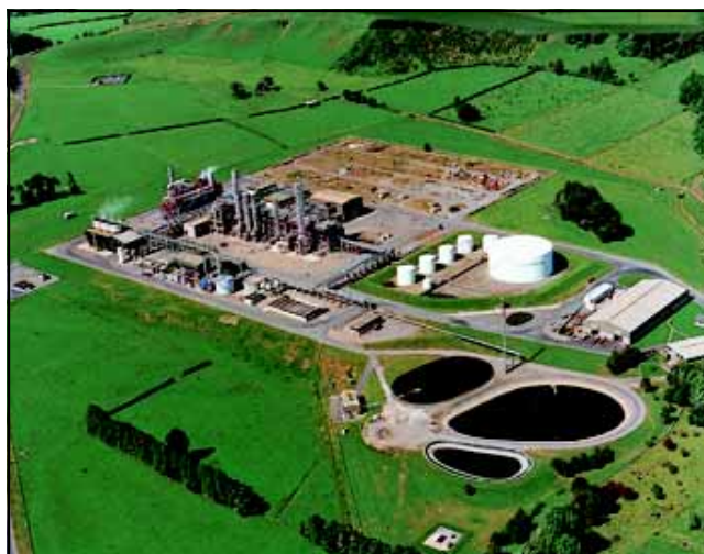
Waitara Valley methanol plant.
