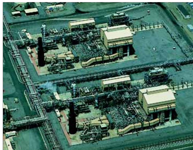
Twin crude methanol units at Methanex's Motunui plant.
