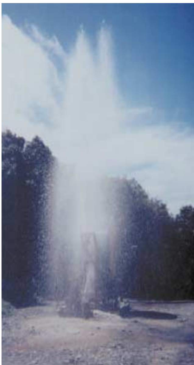
Figure 11: Photograph showing the vigorous ejection of water from the Rapahoe 1 well after water level was drawn down to 160m.
