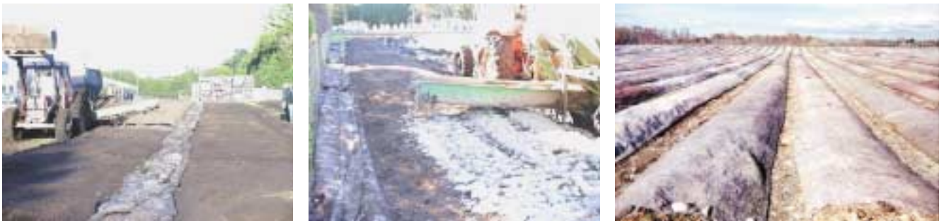
Figure 13: a) and b); Feed out of the blended cuttings and Paunch material onto the worm beds; c) windrow worm beds showing the felt and polypropylene backed covers.
