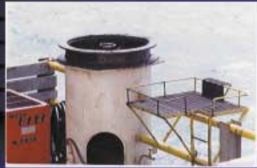
Loss of crane from pedestal - drillship
