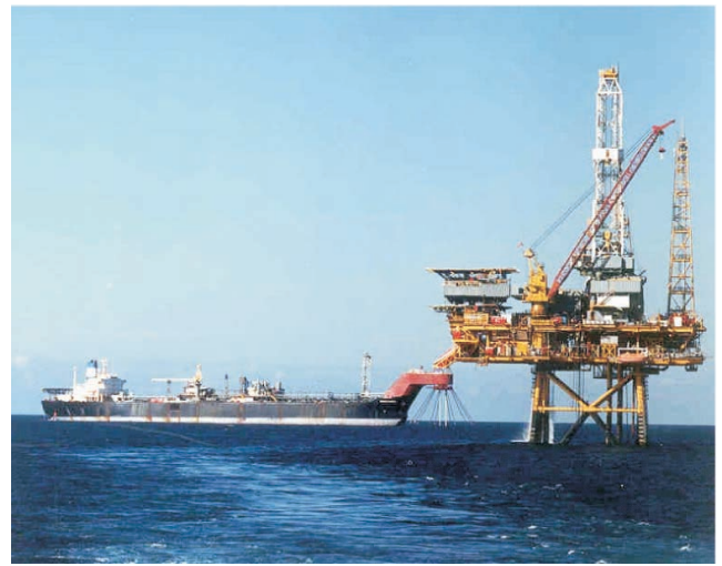
FPSO Installed and on location and Maui B
