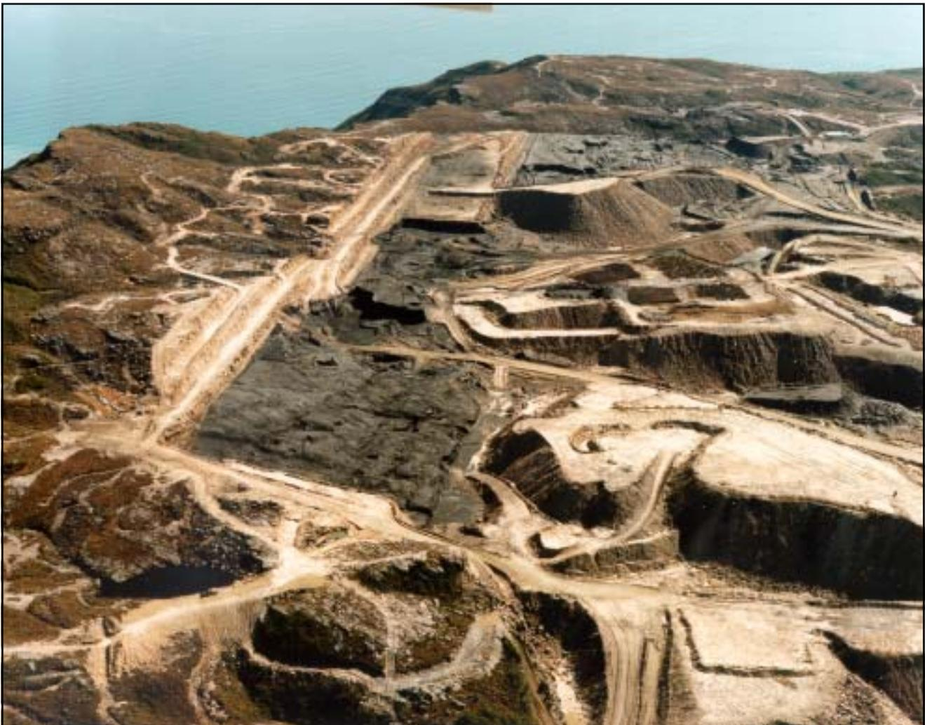
Figure 11: Solid Energy's Webb opencast mine at Stockton in the Buller Coalfield. The mine produces high-quality bituminous coal from a single thick seam near the base of the Brunner Coal Measures (photo: Lloyd Homer).
