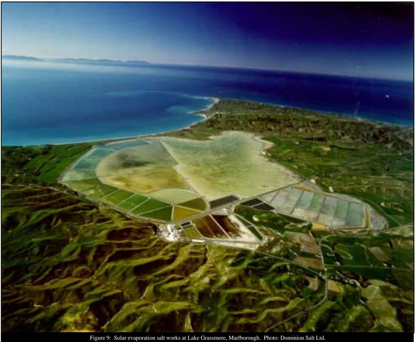
Figure 9: Solar evaporation salt works at Lake Grassmere, Marlborough. Photo: Dominion Salt Ltd.
