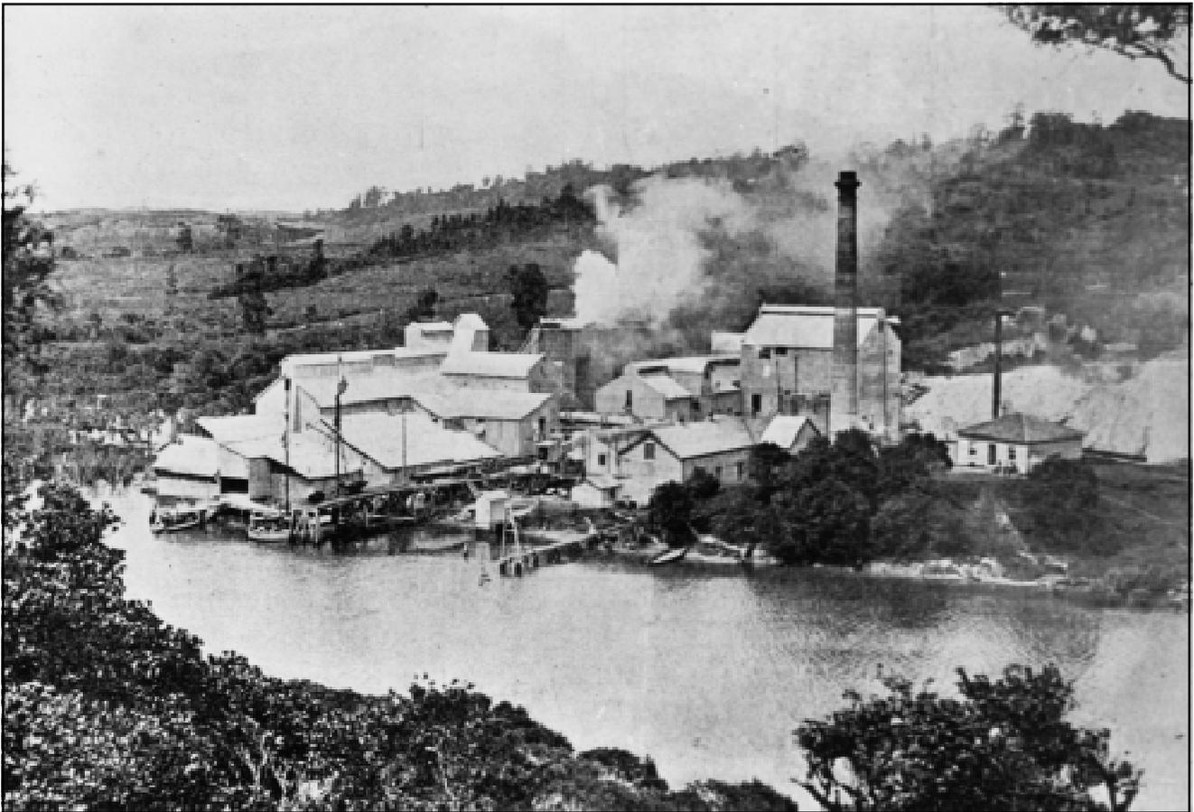
Figure 7: New Zealand's first cement plant at Warkworth in the 1890s with the vertical kilns at the centre of the photo. All product was dispatched in 100 lb sacks in coastal vessels. Photo: Alexander Turnbull Library F118157.5.
